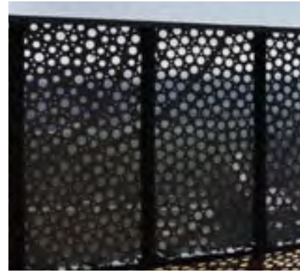
PERFORATED METAL - GUARDRAIL & INFILL PANEL
